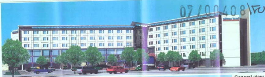
General view of entrance approach from south
