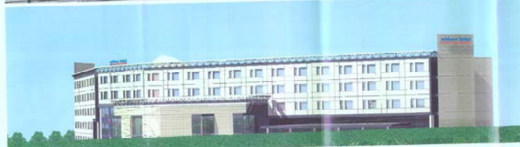
General view from Queensway flyover looking south
